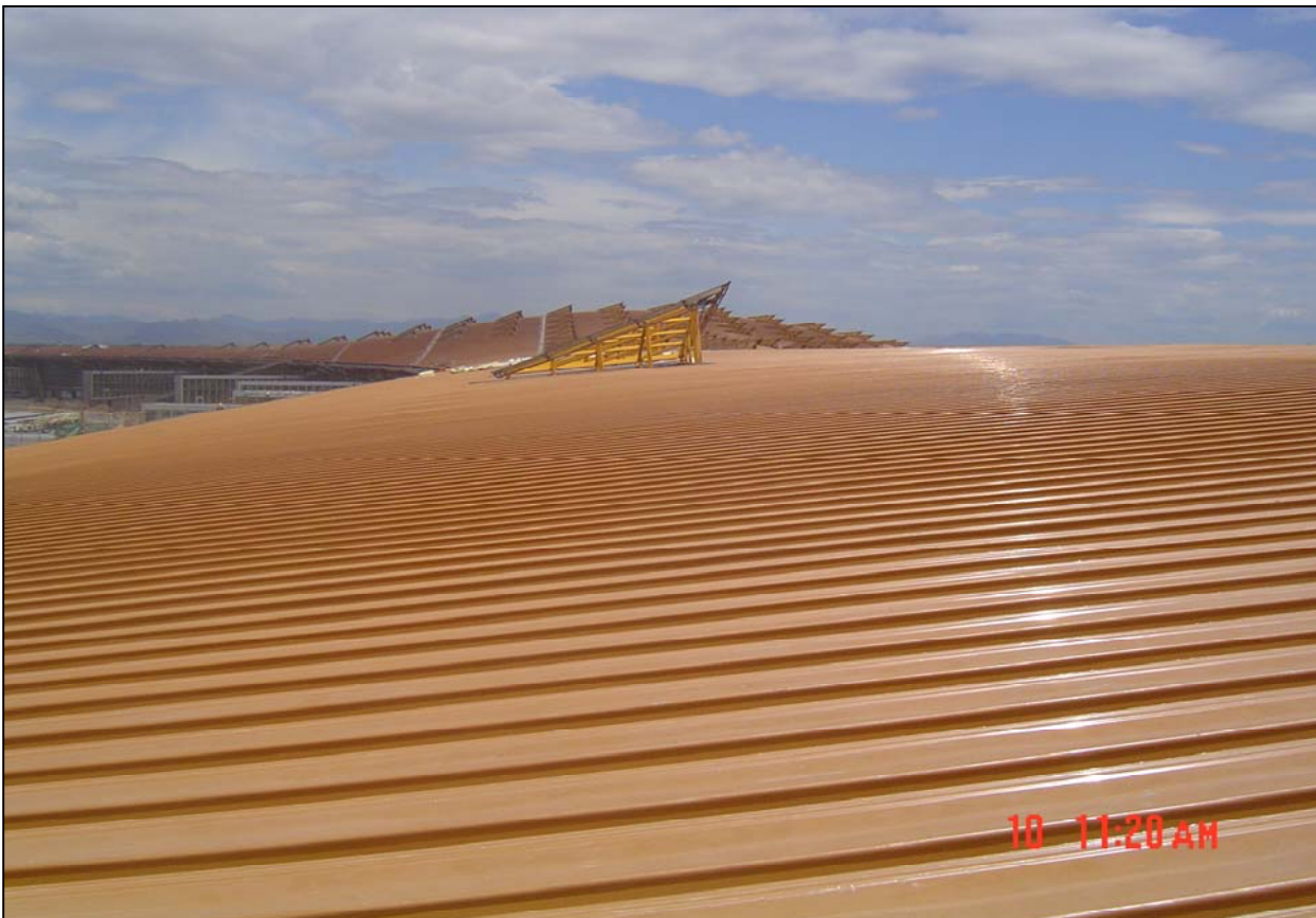
BEIJING CAPITAL AIRPORT TERMINAL BUILDING 3 - STANDING SEAM ROOF 0.9MM HYDRO PVDF COATED ALUMINIUM COIL
